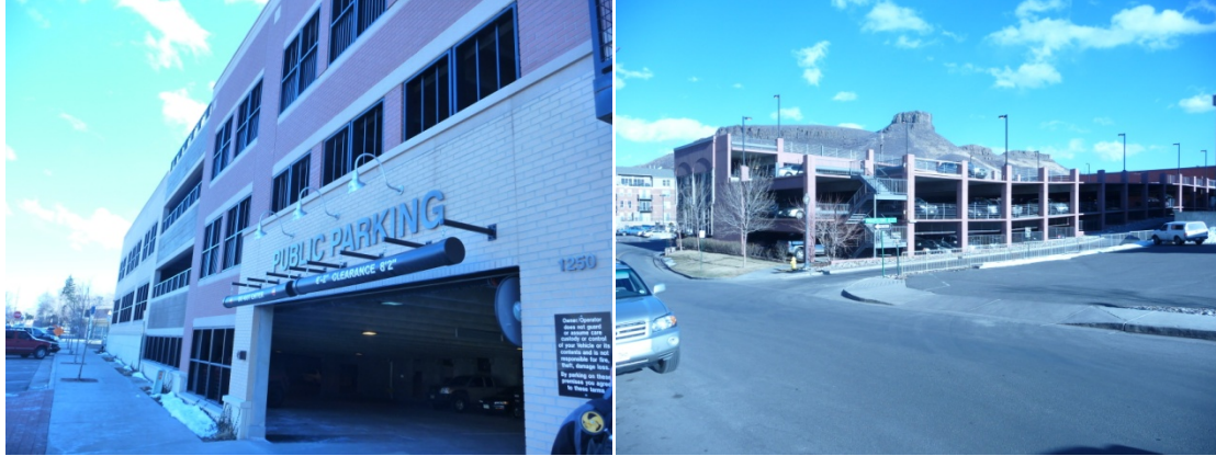
Fig 1: Entry to the Gateway Station Garage Fig 2: Backside of Clear Creek Garage
